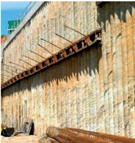
CFA Piles (secant pile wall) for earth retention application and guide wall for CFA piles, Ref: Martin D. Larisch
