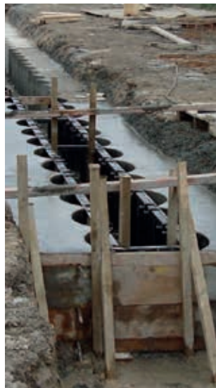
CFA Piles (secant pile wall) for earth retention application and guide wall for CFA piles, Ref: Martin D. Larisch
