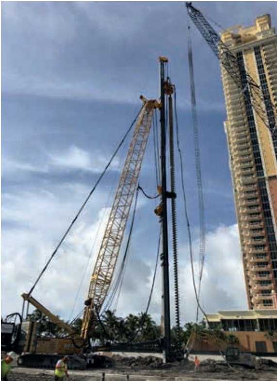
Courtesy; Keller: 760mm to 910mm x 55m (Special case) - HJ Foundation - World Record
