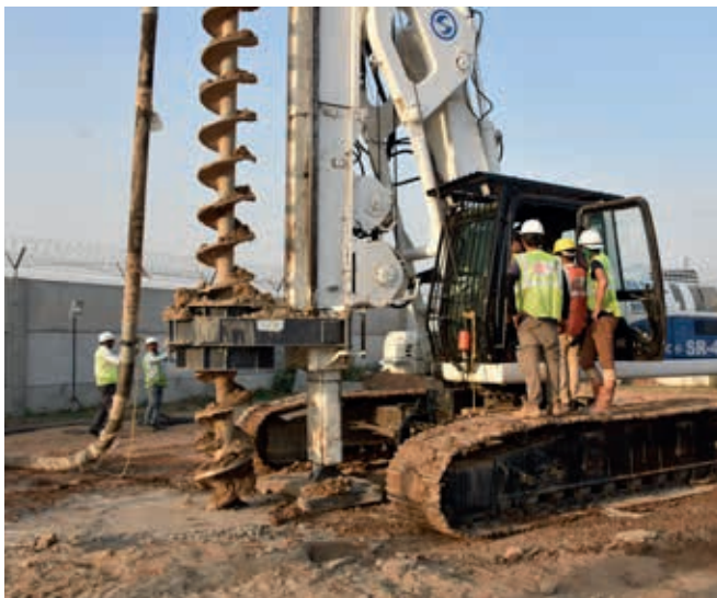
Pile boring in progress using CFA
