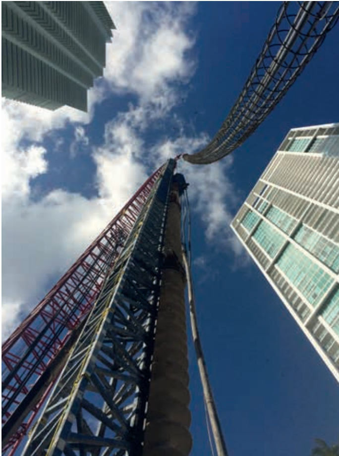
Courtesy; Keller: 760mm x 54m - ACIP-HJ Foundation - Full Length Reinforcing - One Thousand Museum in Miami.
