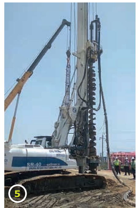
1) RMC truck and concrete, 2) grout / concrete pumping unit, 3) Automated Monitoring Unit installed within rig panel 4) grout / concrete hose, 5) Piling with hydraulic rotary rig mounted continuous flight auger and long boom crane
