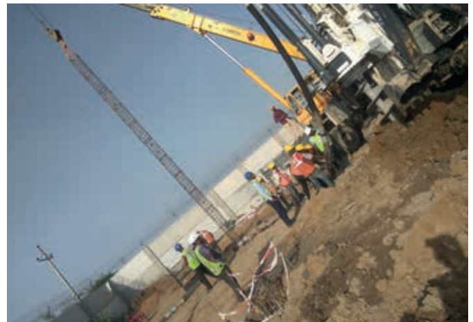
Pile boring in progress using CFA
