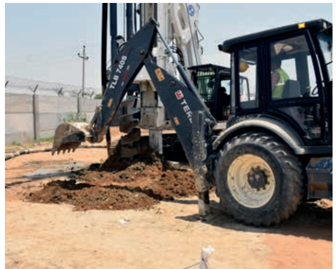
Muck removal around pile by Excavator
