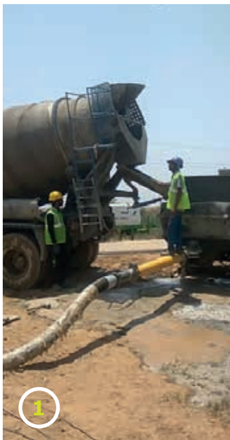
1) RMC truck and concrete, 2) grout / concrete pumping unit, 3) Automated Monitoring Unit installed within rig panel 4) grout / concrete hose, 5) Piling with hydraulic rotary rig mounted continuous flight auger and long boom crane
